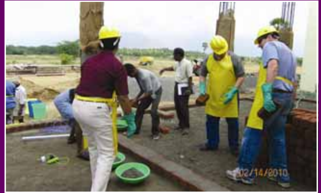
Building on to a school at Rajapalayam
